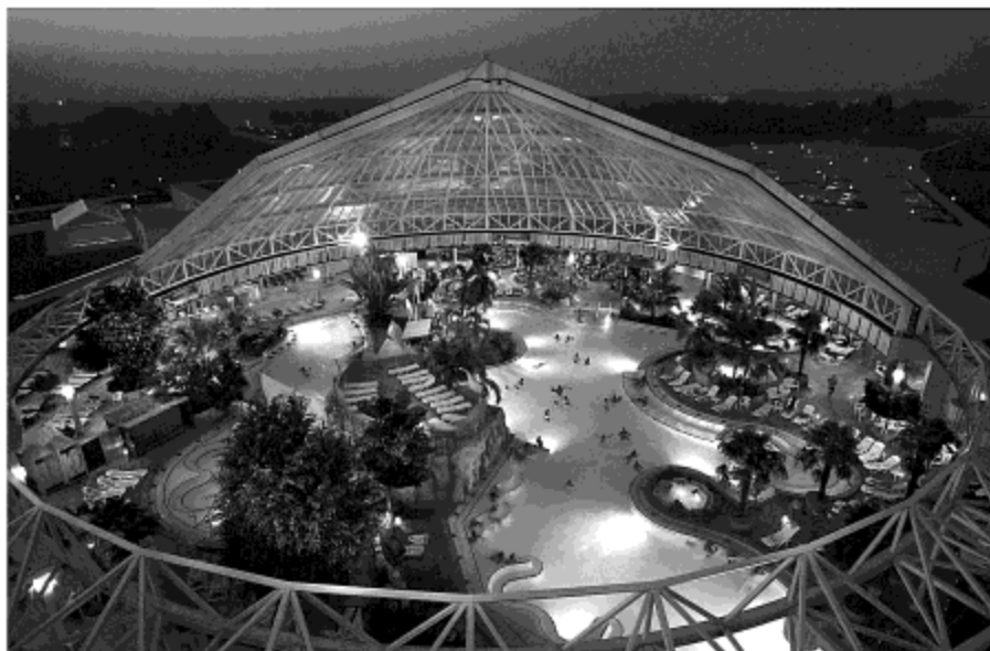
Overview of the enormous thermal bath and spa complex Therme Erding
